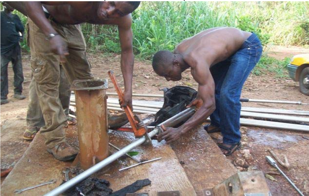
Project in process.
